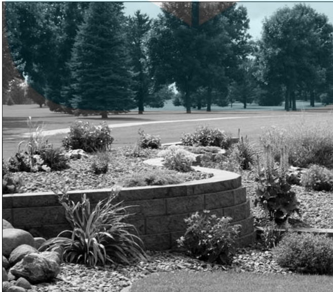
Figure 12-1: A segmental retaining wall.
